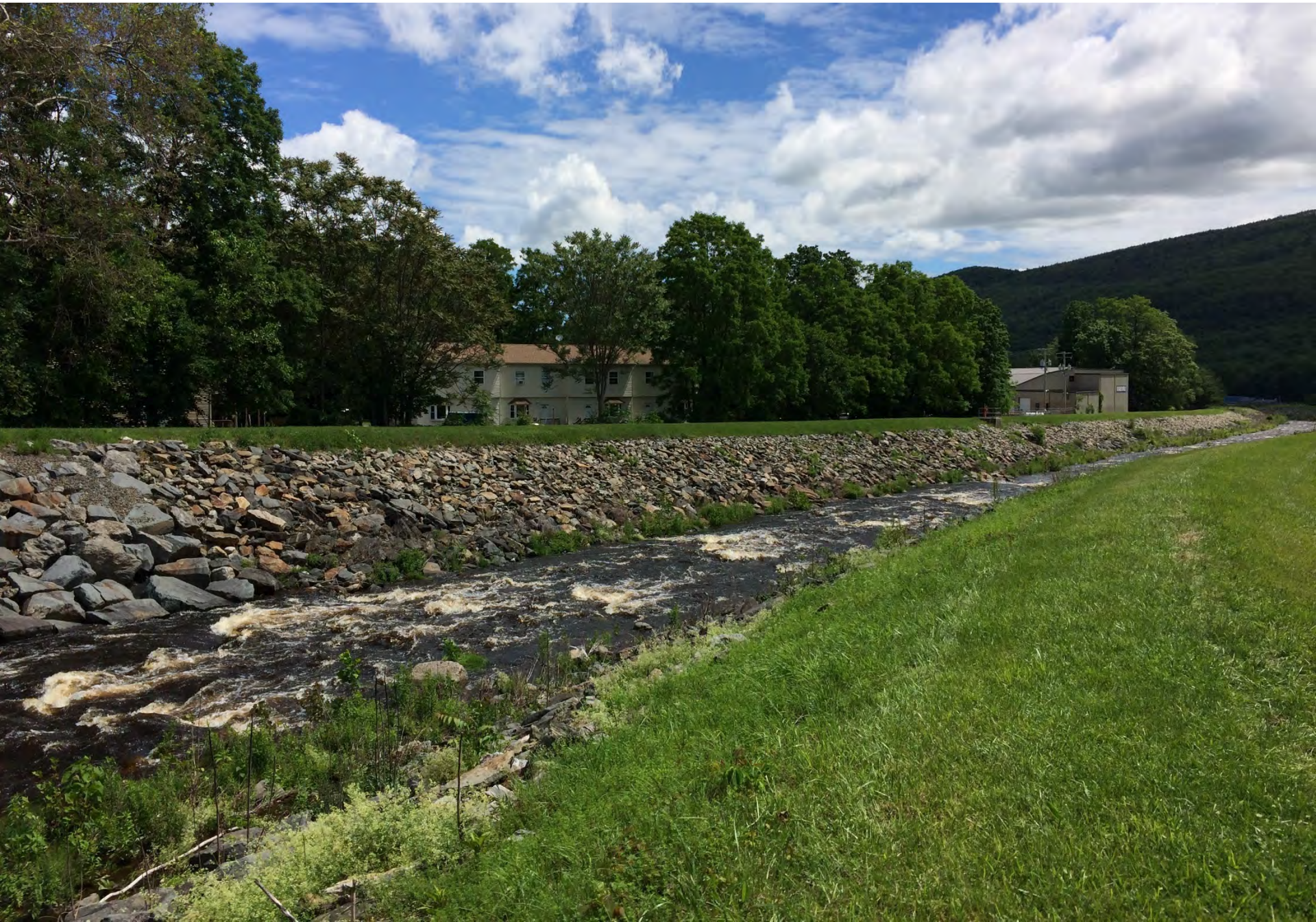
Beer Kill Left and Right Bank Levees Looking East from Just Downstream of Main Street
