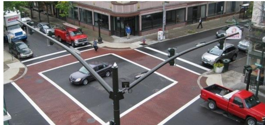
ITS Signal Improvements, Troy
