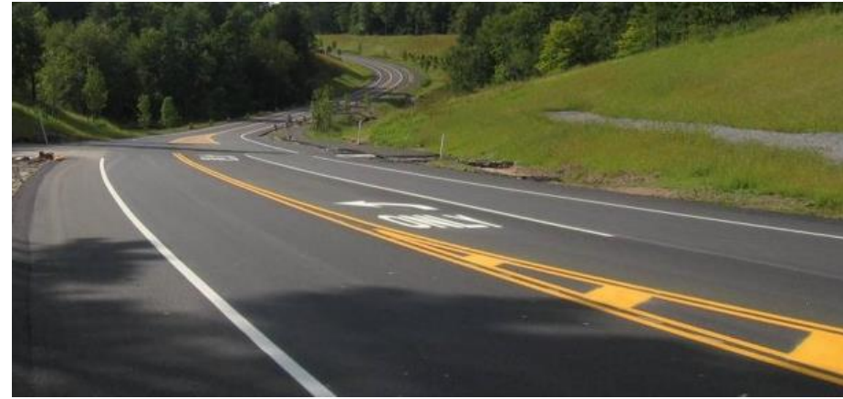
Luther Forest Technology Campus Roads, Malta
