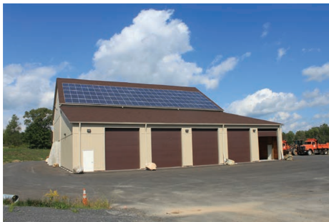
In 2010, Ulster County installed its first renewable energy system at the New Paltz Highway Substation. This 30.6 kw PV system is located "behind the meter" at the substation.
